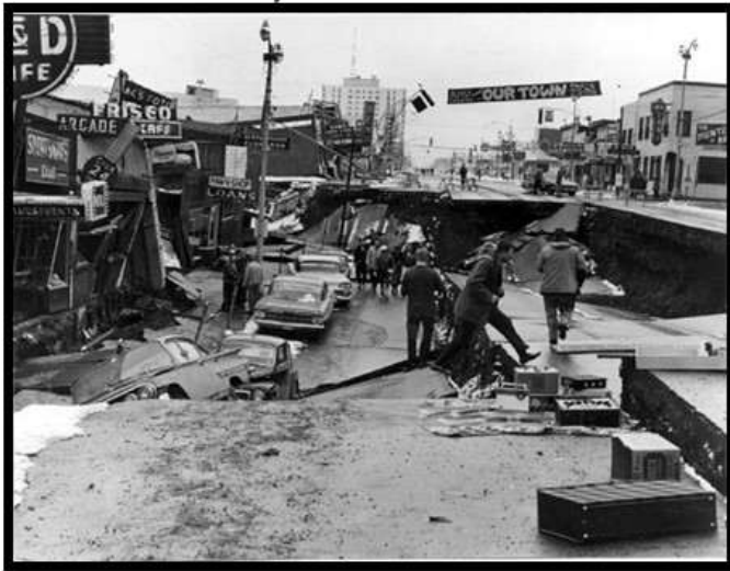
Collapse of Fourth Avenue near C Street, Anchorage, due to earthquake caused landslide. Anchorage district, Cook Inlet region, Alaska. 1964.
